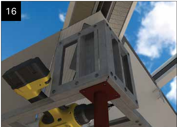
Valley infill panel fitted to horizontal frame, as image 10.
