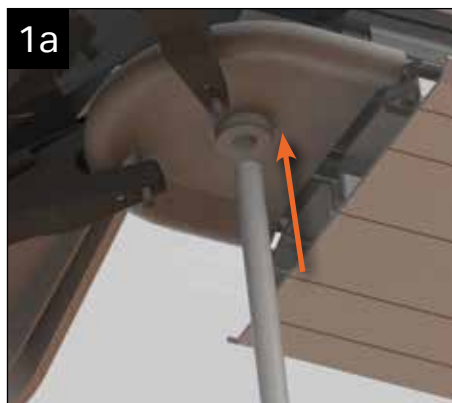
Tie bar at finial Insert the tie steel rod thread into the base of the spider. Measure the drop of the rod and cut to suit the position or the tie bar boss ring.
