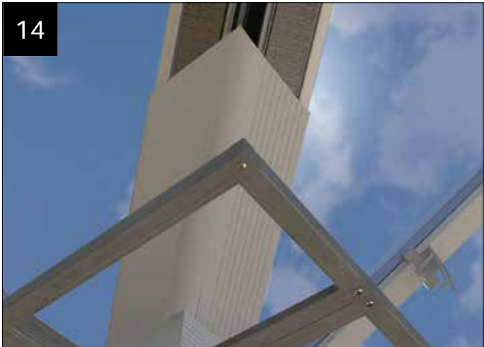
Measure and fit the standard valley undercladding NVU-V between the eaves and mark 'C'. Scribe to suit.
